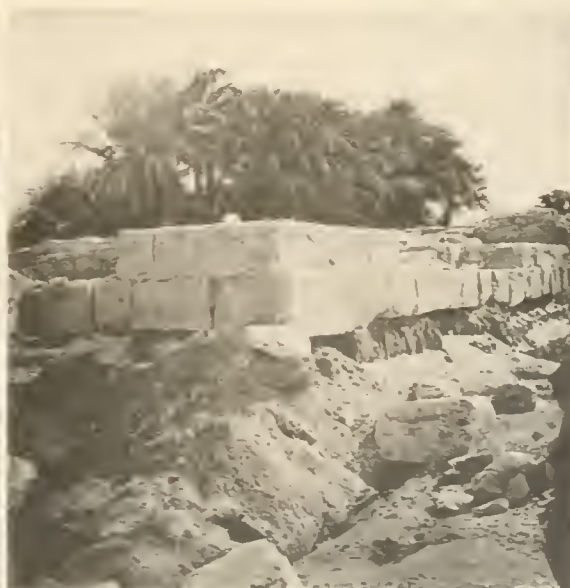
6. FOUNDATIONS OF AAHMES II.
